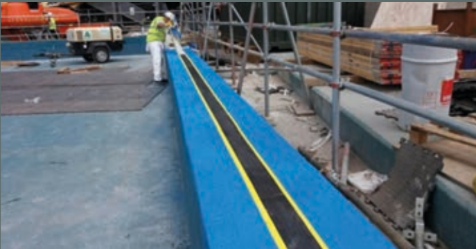
Above: Blueshield PmB lapped onto Migupren to ensure complete waterproofing integrity
