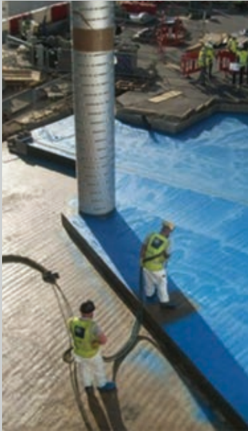
Above: Operatives applying Blueshield PmB to the concourse using sophisticated spray technology
